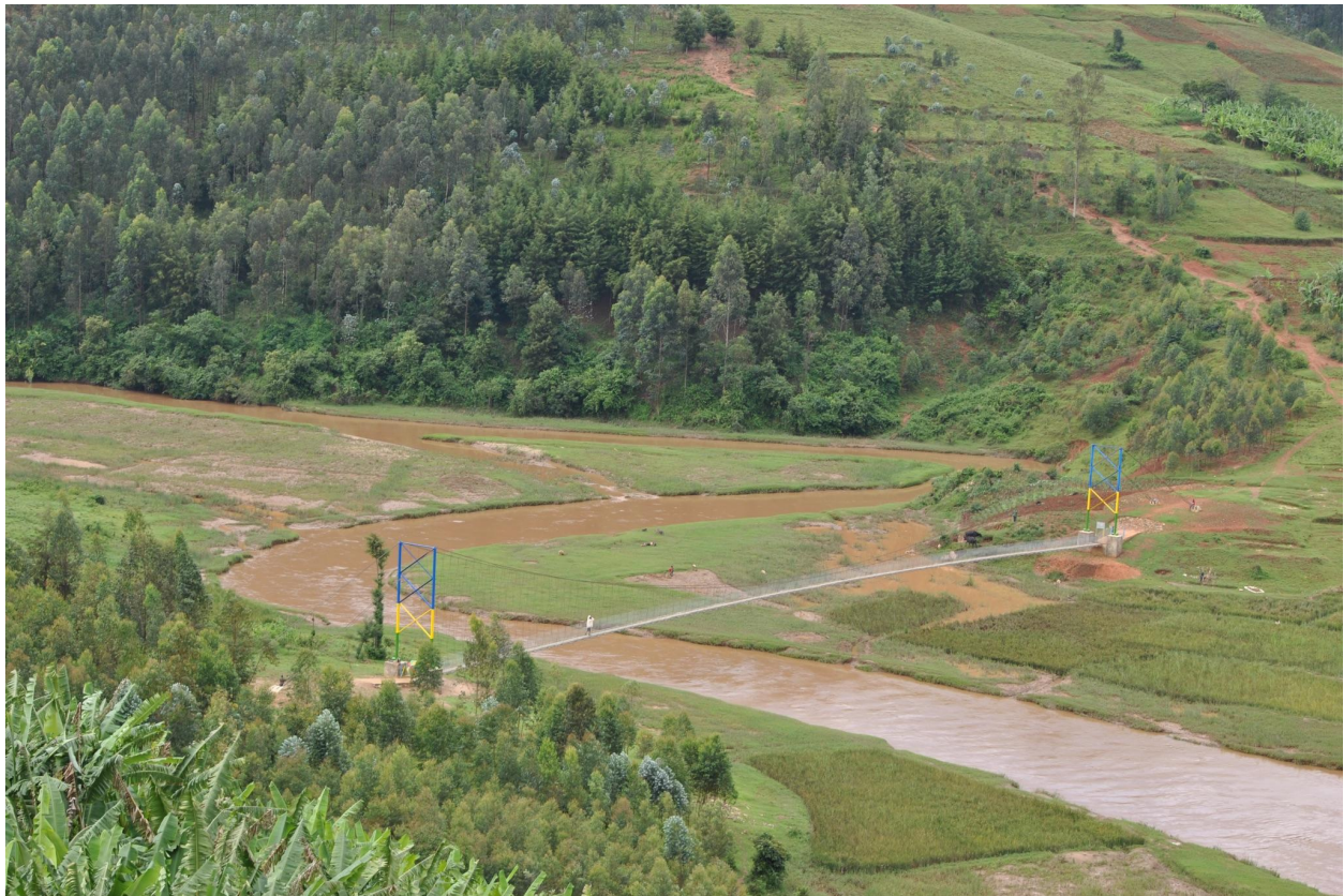
Photograph 1: A photograph of the Nyakabuye-Mwogo suspension bridge, completed October 6, 2020 in Rwanda.
