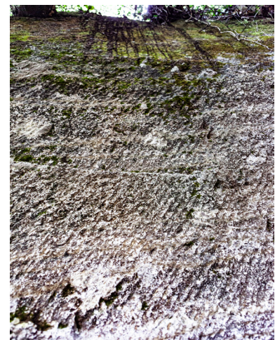
Fig. 1 and 2. Author: Elena Lavellés. Photographs of the quarries of Tusculum. The city of Tusculum was one of the largest and oldest in Italy. In its quarries you can still see the marks of the tools left more than two thousand years ago by the workers when extracting the stone blocks.
