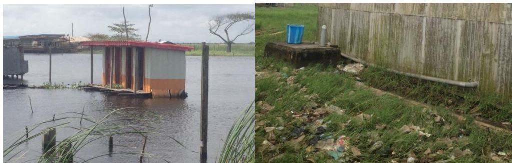
Figure 2: a) Pit Latrine b) Septic Tank of flush toilet
