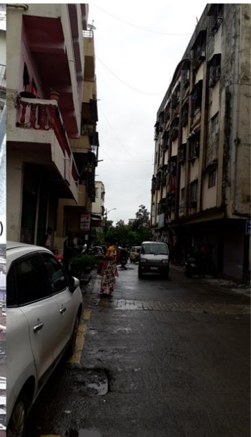
Fig 6 Unmaintained buildings (Group C)
