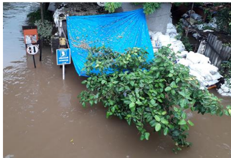
Fig 4 Community Toilet in flood waters
