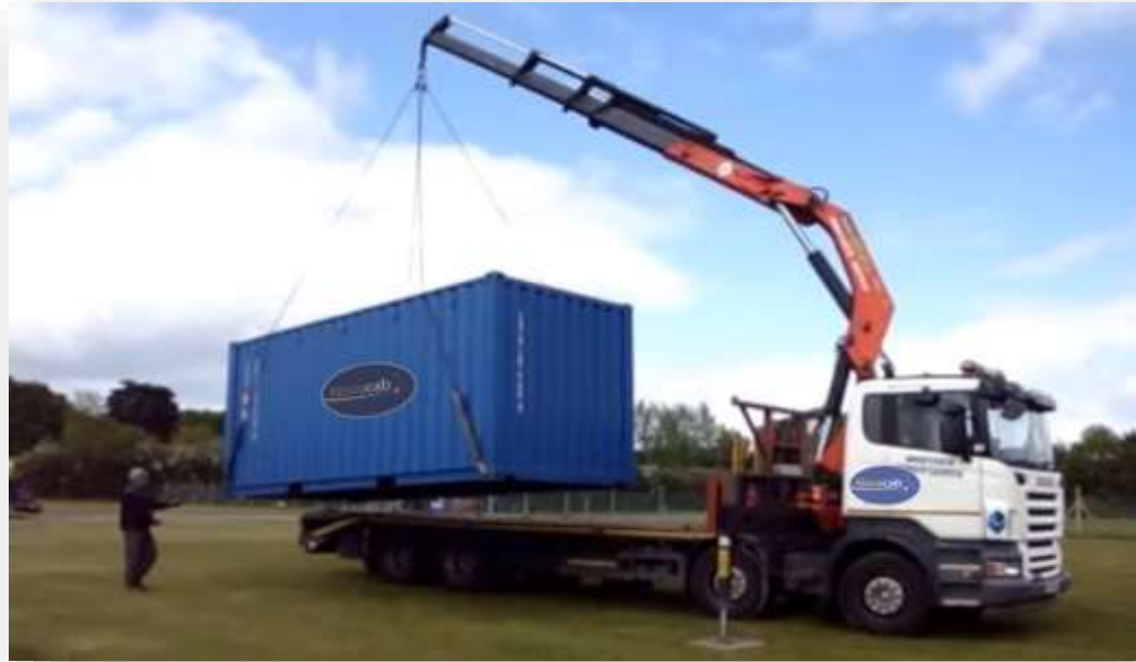
Fig. 3. Thermal/electrical energy storage unit being delivered
