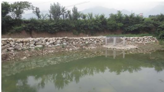
Figure 3: *Laochi* under construction with a stone dam in Heiyu Village, Meixian County
