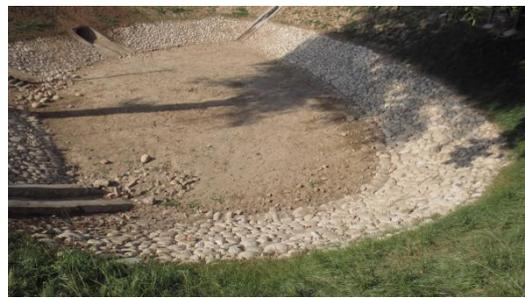
Figure 4: *Laochi* under construction with a stone layer in Xiaoqiang Village, Qishan County
